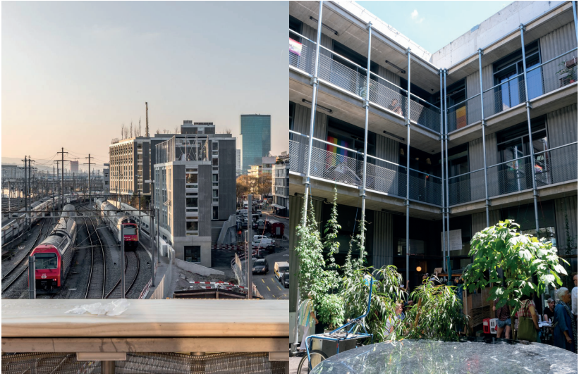
30 Left: The Zollhaus next to the traintracks
