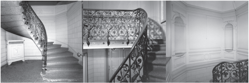
10 Left: The Staircase in the extension with ashlar masonry in the base, 1989
